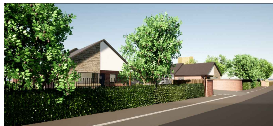
View along frontage to Melton Road.
